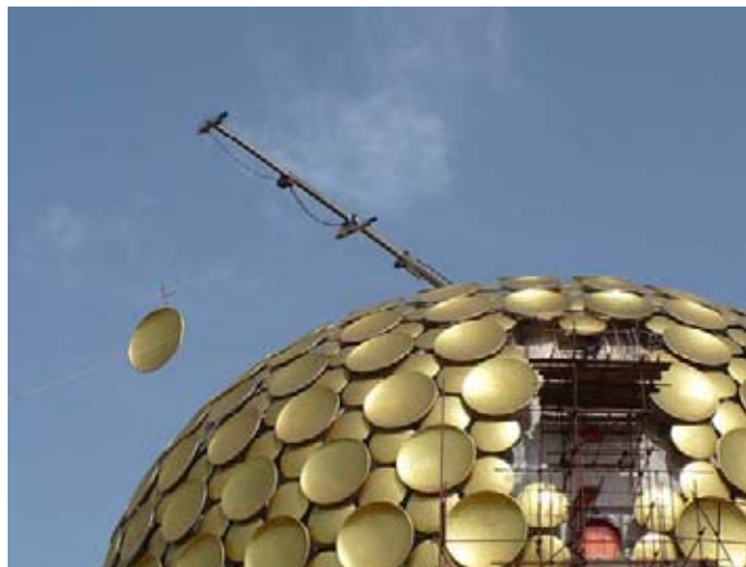
The new Matrimandir crane lifting a disc
